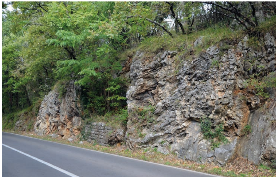
Fig. 11.22: Crushed limestone in the inner Divača Fault zone at Stop 7 (Photo: M. Novak)
